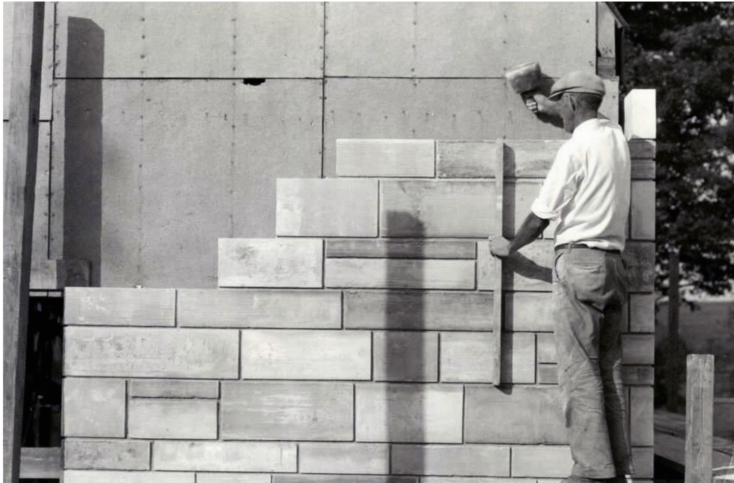
A mason installing an Indiana Limestone full-bed veneer wall in 1929.
