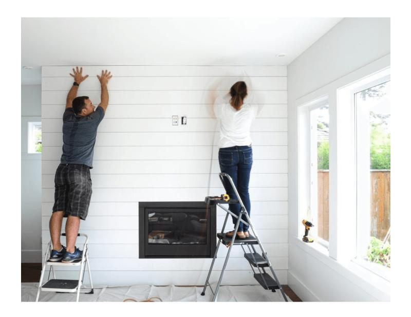
While you're installing your shiplap, you want to ensure that there's a 1/8" gap between boards and that every nail is hidden. To hide them, you should nail them into the dado of each plank.
